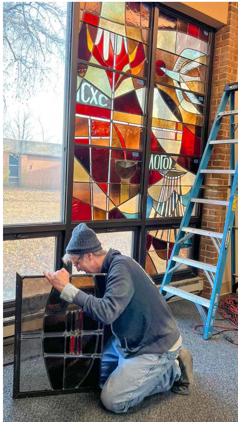
A craftsman from the Emil Frei Company removes the stained glass windows from the province center chapel.
